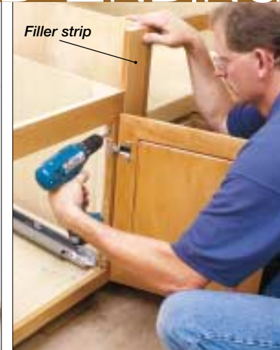
Filler strips are ripped to the required width and attached to the face frame of neighboring cabinets in the same way you connect two units, as shown in the "Making Connections" photos, p. 31.
