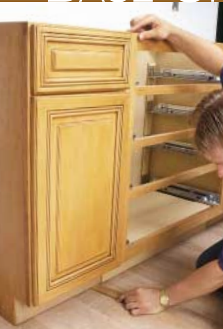
Insert shims as needed to level cabinets along the front and back edges. Be sure all units are supported at their corners.
