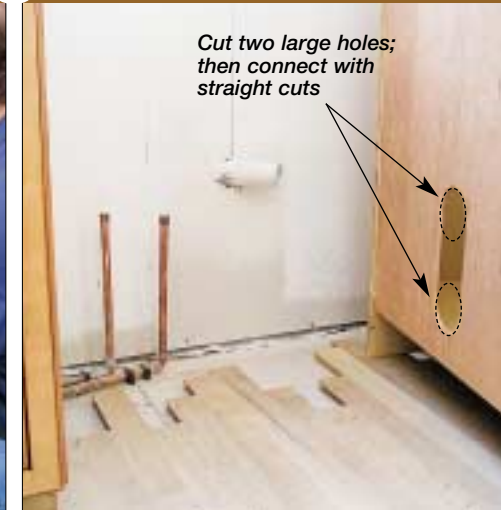
To mark locations of pipes, measure horizontal distances along the wall from the edge of the neighboring unit. For easier transfer of dimensions, keep the sink base close to the wall as you measure and mark.
